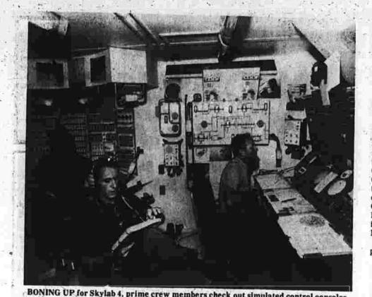
BONING UP for Skylab 4, prime crew members check out simulated control consoles at Houston's Johnson Space Center. Mission commander Gerald P. Carr, right, is seated at the control and display console for the Apollo Telescope Mount which is lo-cated in the space station's Multiple Docking Adapter. At left is scientist-astronaut Edward C. Gibson and at left background, Skylab 4 pilot William R. Pogue.
